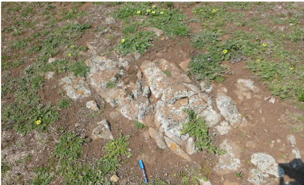
Photo 7: View looking at bedrock exposed near the crest of the steep to very steep hillside near the small water reservoir in the northern part of the site.
